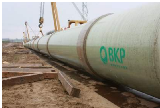
Steelpipe protection (horizontal drilling, pipe ramming)
